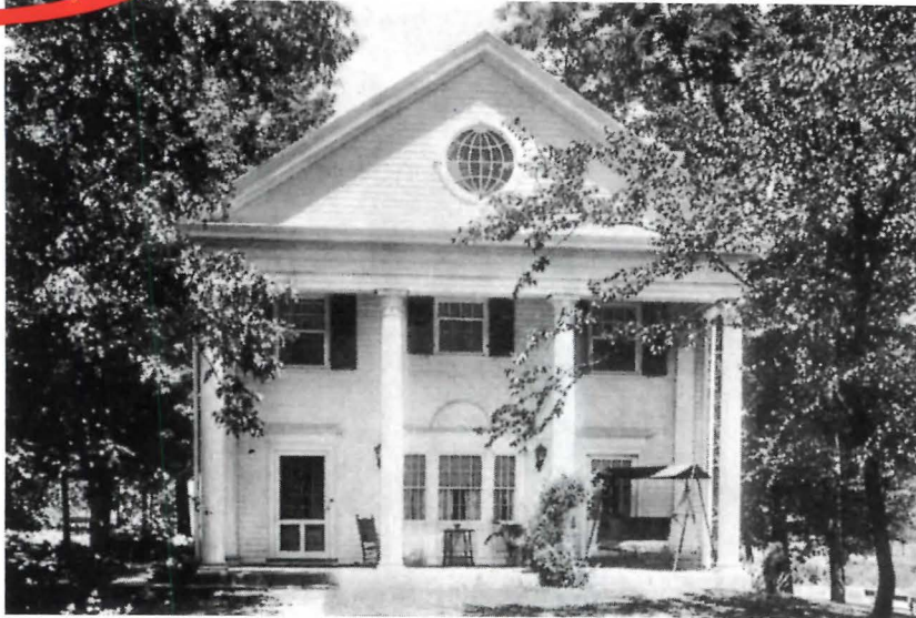
Home of Mr. Walter H. Merritt, Tenafly, N. J. R. C. Hunter & Bro., New York, Architects
