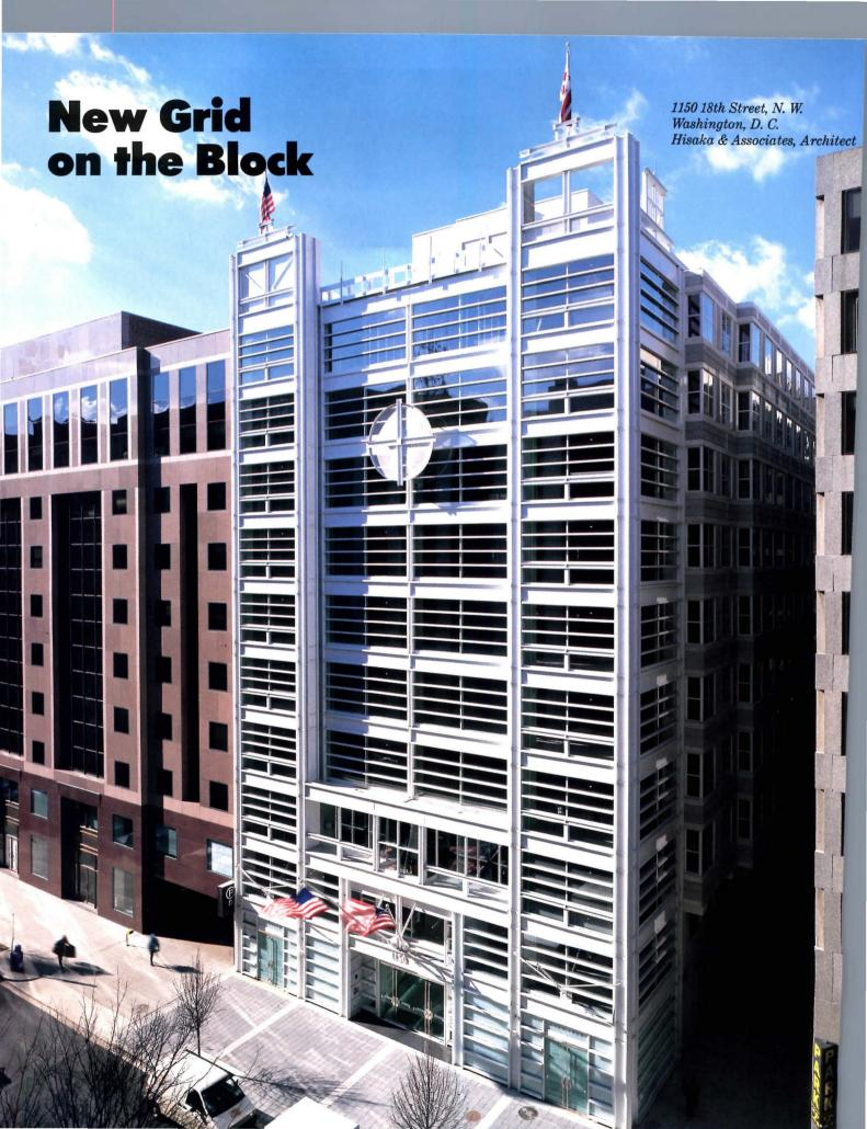
ith its facade dimensions reordained by a 75-foot street ontage and 10-story height nit (plus English basement nd two floors of underground erking), 1150 18th Street rns its relatively small size 87,000 square feet with 17,000uare-foot floor plates) to lvantage with a lighthearted rtain wall (opposite) whose ergy would overpower at rger scale. Similarly, the ng angled approach from the reet entrance to the midblock rium/lobby becomes an entful progress through a vely retail arcade.
