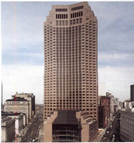
BP America Building, Cleveland, Ohio Architect: Hellmuth, Obata & Kassabaum, Inc. Photo: Bill Schuemann
