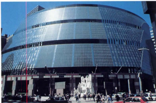
State of Illinois Center
