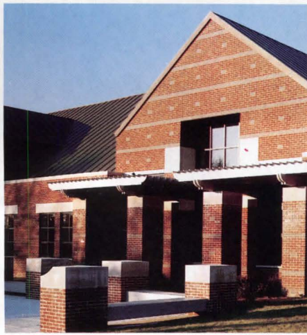
Imperatore Library, Englewood, New Jersey Architect: Bohlin Powell Larkin Cywinski Photo: Christopher Barone
