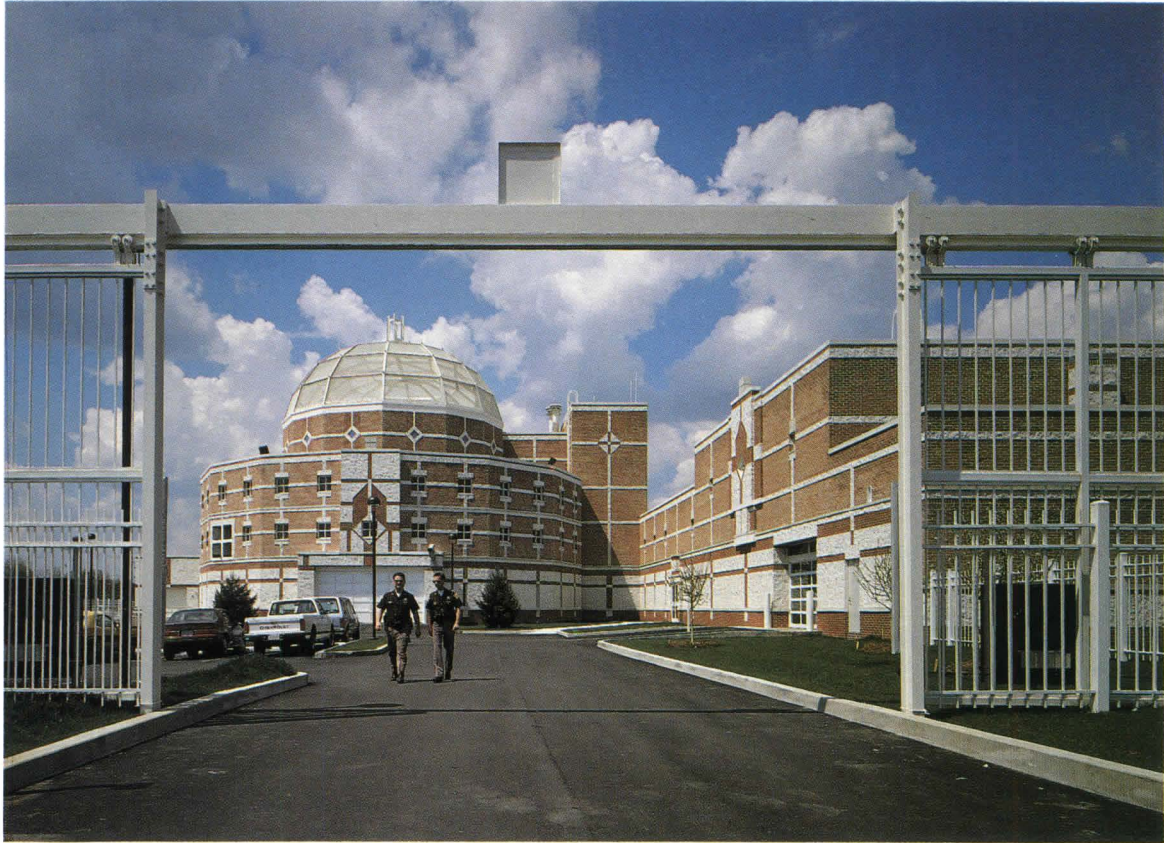
In addition to shielding the jail from public gaze, the two-story support building disguises its bulk. The full-block site that fosters privacy and security also allows addition of another cell-block when needed.
