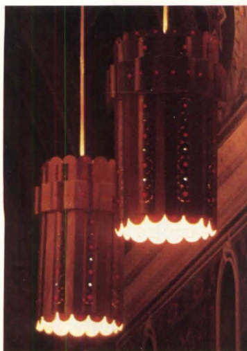
Architects revamped St. Clement's lighting and created bronze chandeliers run by a dimming system (above). Fixtures (below) contain three uplights and one downlight, 500 watts each. Light diffuses through the egg-crate bottom.
