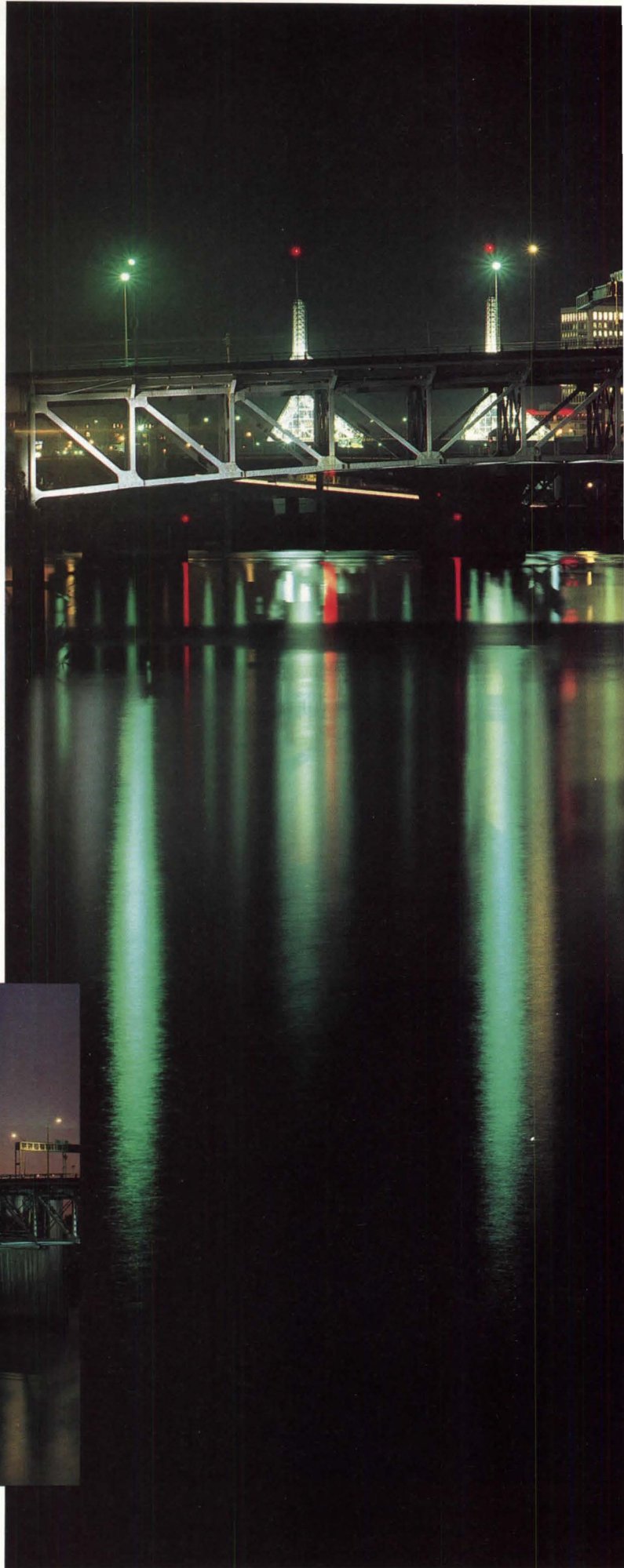
Four floodlights mounted on the piers play on the rugged structure of the Morrison Bridge. Color comes from plastic gels on the luminaires, which are changed periodically.
