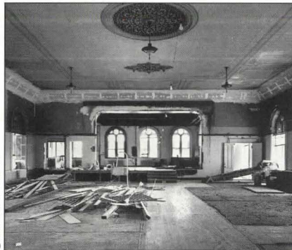
The auditorium before $2.1-million restoration.
