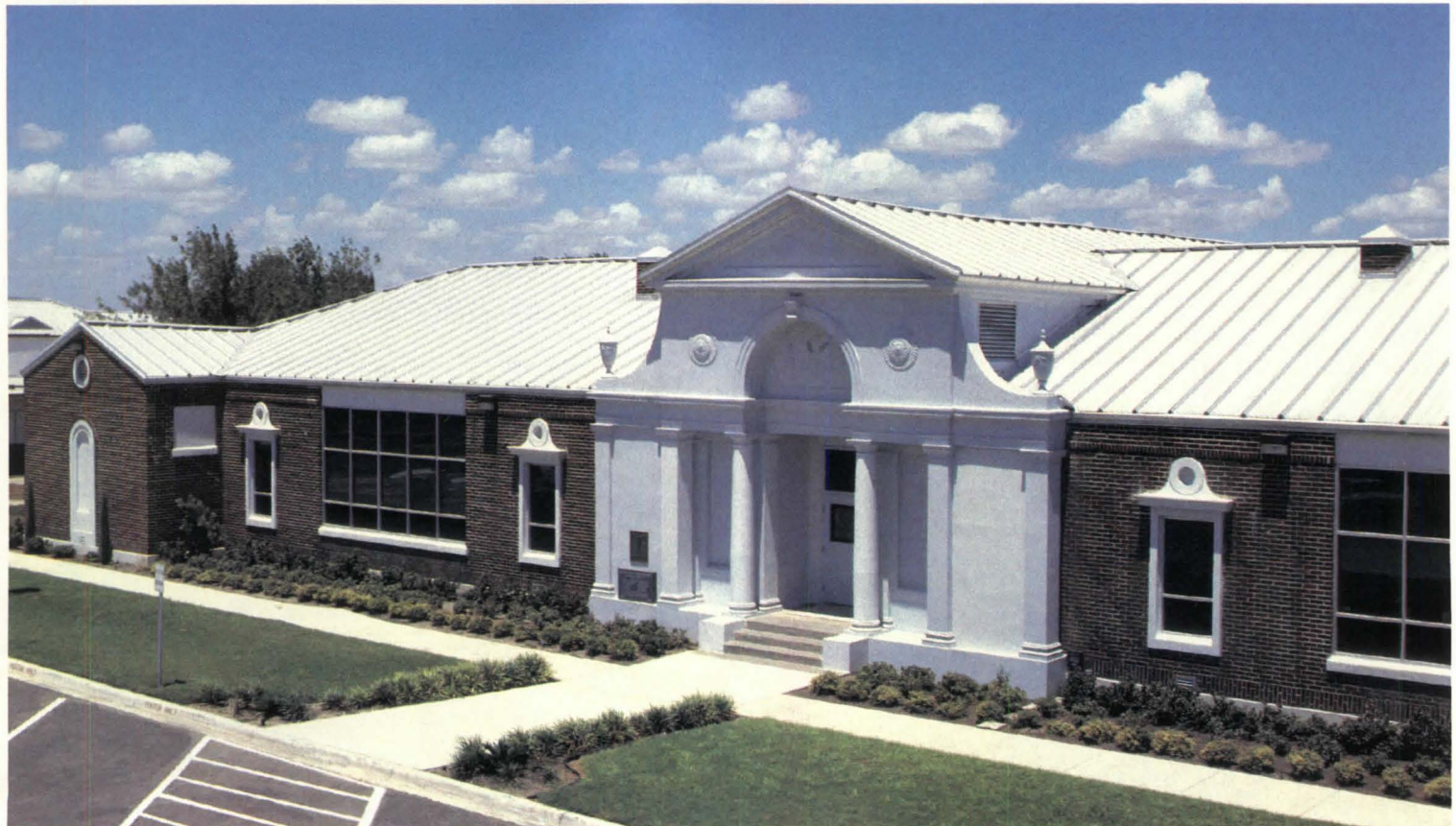
Project: Sharyland I.S.D. Administration Building Renovation Architect: Boultinghouse, Bustos & Associates Roofing Contractor: Bullard Sheet Metal & Roofing Co. Roofing Material: MBCI's Standing Seam Ultra-Dek 124® , Bare Galvalume
