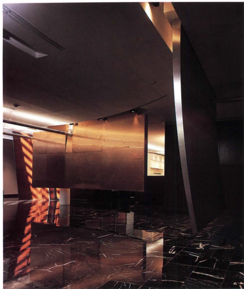
Curved metal partitions hang from the ceiling.
