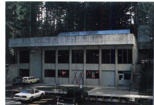
Miller/Hull's new studio building (left in top photo) is linked to the original building (small photo above) by a generous lobby/gathering space.
