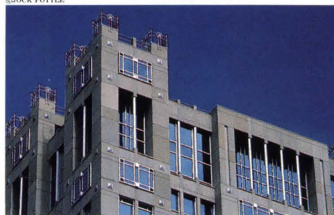
Top: light fixture in the mall of 900 North Michigan Avenue. Bottom: the crown of 101 Federal Street.
