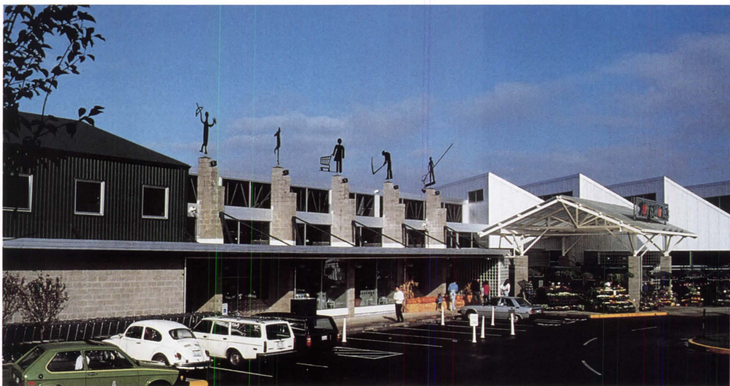
Larry's Market Kirkland, Washington Carlson/Ferrin Architects
