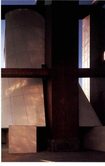
As a result, the siding looks as if it has been quilted, and its billowy patches seem to breathe air into the oversized sheds. Dominating the complex is a 70-foot-high copper trellis stitched together with steel bolts. This open network encases a conical skylit employee cafeteria (above right and opposite page) and frames an alluring composite of construction details and land-scape still-lifes that shifts as visitors move across the concrete courtyard.
