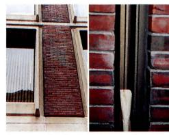
An example of a location requiring a fillet joint (left) and application of new sealant over old (right).
