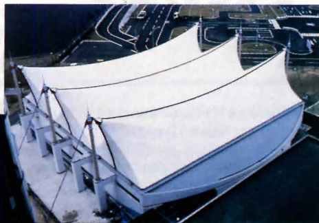
Point-hung tensioned membrane structure at Toyohashi.
