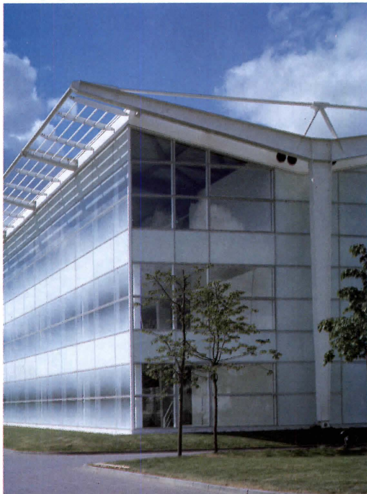
Building B3, Stockley Park
