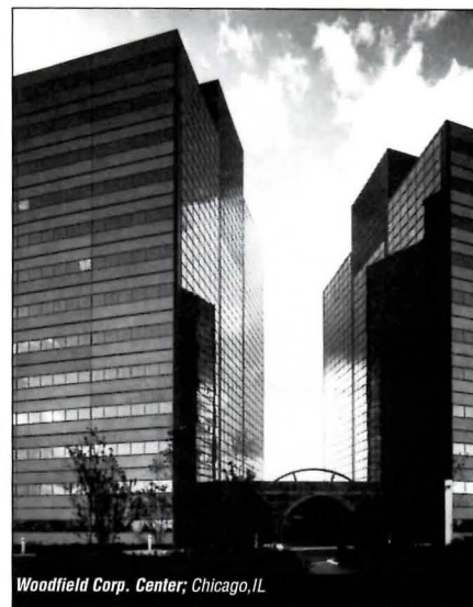
Woodfield Corp. Center, Chicago, IL Arch: Holabird-Rood • Cont: Popper Const. Co. • Erector: Engineered Erection Co., Inc.
