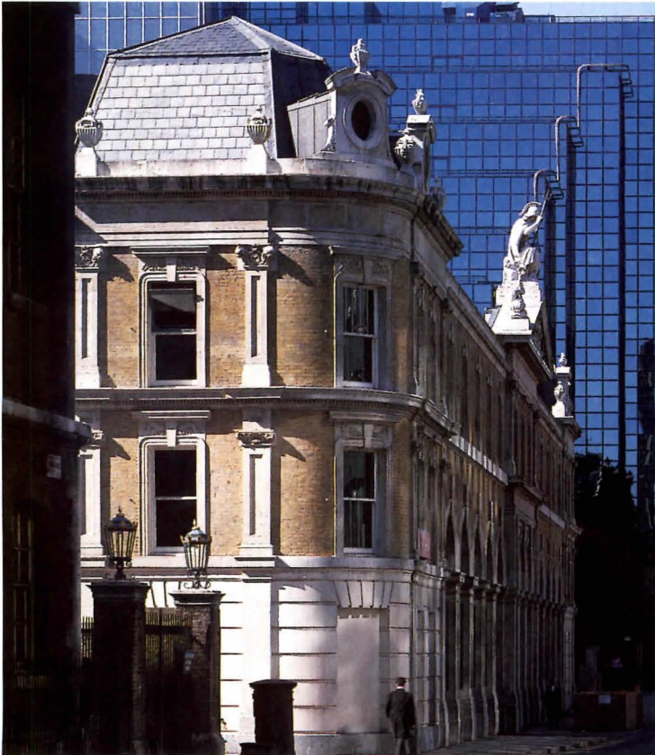
The Richard Rogers Partnership's sensitive renovation of the Thameside Billingsgate Market into offices for Citicorp called for cleaning and repairing Horace Jones's 1875 masonry exterior (above), including a fish-topped weathervane (top).
