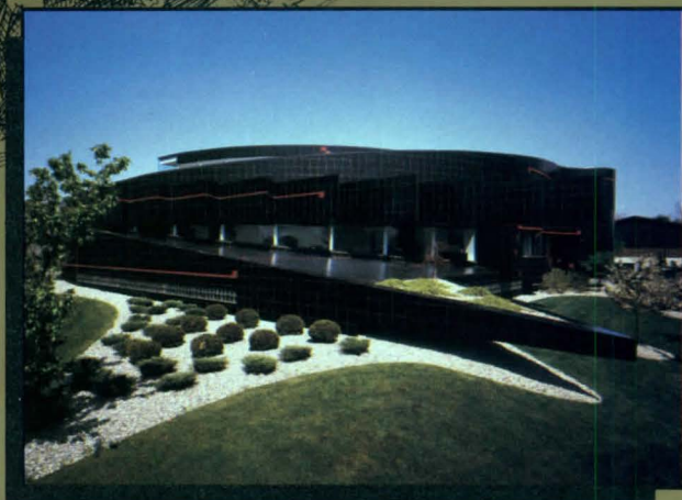
Architect: Harvey Ferrero Roofing Contractor: Brodak Roofing & Sheet Metal Carlisle Manufacturer's Representative: Holmes Associates
