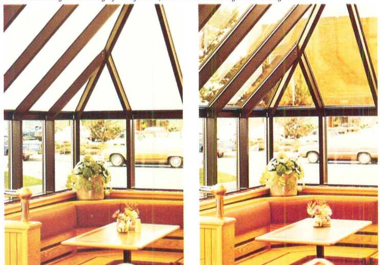
Sloped glazing in the illustrated café shows the off (right photo) and on characteristics of "switchable" glazing. The glass is coated with a flexible polymer film encapsulating tiny spheres of liquid crystals. The liquid
