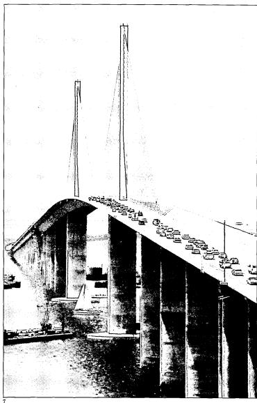
7. Sunshine Skyway Bridge, Tampa Bay, Fla.; Figg and Muller Engineers. The 1,200-ft main span is the longest of any concrete cable-stayed bridge in the U.S. Sections of the roadway were precast on site and then placed in their final position. Reinforcing steel was epoxycovered to retard corrosion in the severe marine environment. The jury exclaimed, "This has to be
