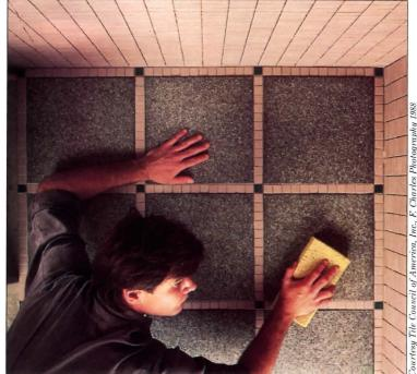
notched trowel of the er depth must be used to e the thickness of the 'ar, combing it into ridges circular pattern. (2) After is set in place with a ing motion to align it with s, it is beaten into the ar, which compresses the
