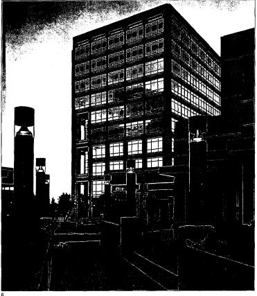
5. Student Services Building, University of Utah, Salt Lake City; Astle/Ericson & Associates, Architects. Reinforced concrete was initially employed to reduce the floor-tofloor height, permitting connection to an adjacent historic building. The jury was impressed by the articulation of the structural elements, which took idvantage of "the strong nherent visual characteristics of einforced concrete." In addition, the inventive control of light 'creates a very warm structure."
