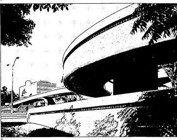
1. The Terraces at Perimeter Center, Atlanta; Skidmore, Owings & Merrill, Architects. The glass curtain wall is progressively set back from the exposed poured-in-place frame at the highest floors of these office buildings, creating the balconies referred to in the project's name. The jury found the project to be "very comfortable for Atlanta," and hailed "the coherence of all the parts... and the very fine workmanship."
