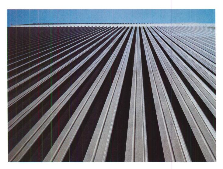
On and on and on. For as long as 150 feet without stopping. That's the beauty of Cot-R-Cap<sup>®</sup> exterior surfacing. Its patented construction offers continuous battens and panels that keep going. Even over ridges and other direction changes.
