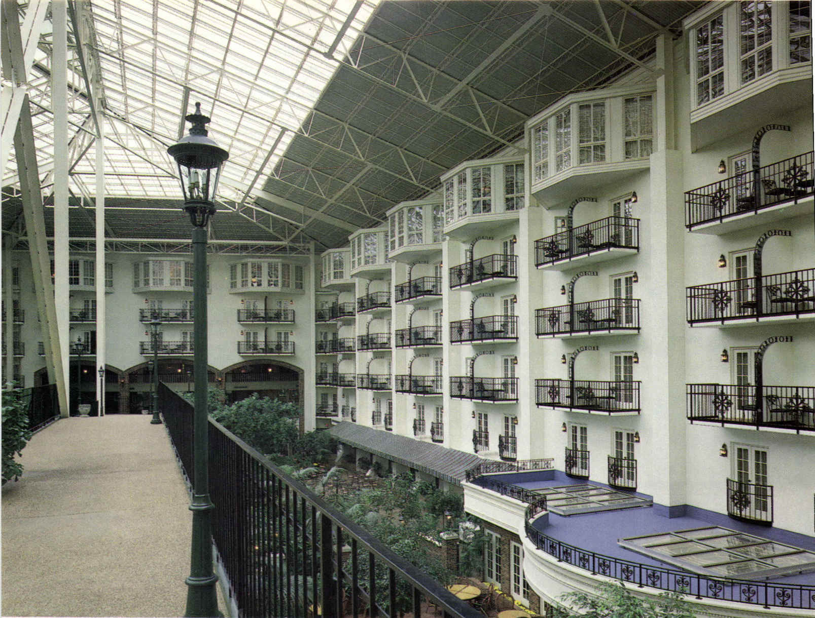
At the pinnacle of the Opryland Hotel Conservatory's lush indoor Victorian garden are angle bay windows, custom built for the hotel.
