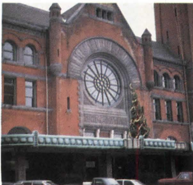
Union Station, Indianapolis
