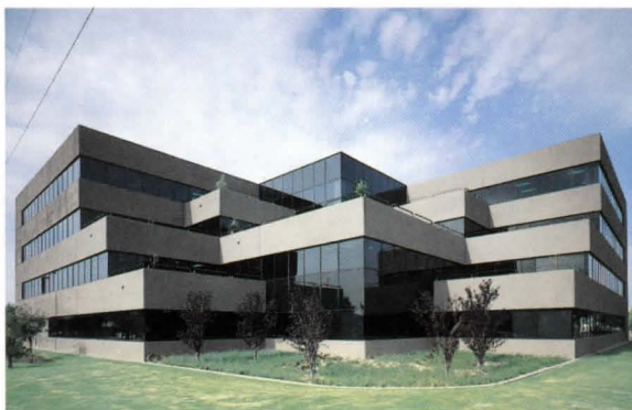
Terra Office Building, Phoenix
