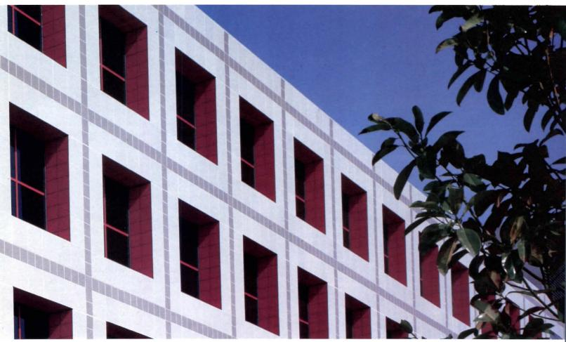
Exterior ceramic cladding. A design statement used by innovative architects to achieve enduring color, proportion, and resistance to weathering.
