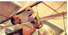
3. Tap is installed at fixture location by aligning terminal block in neutral
