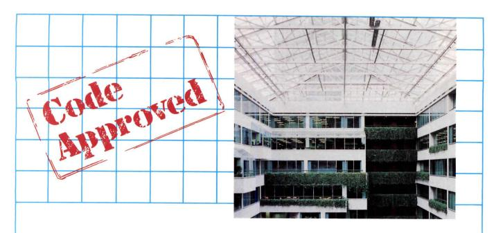
Architects list safety as a primary consideration in overhead glazing design. That is why laminated safety glass was specified in atrium of the Philadelphia Stock Exchange. In the event of breakage, laminated glass tends to remain
