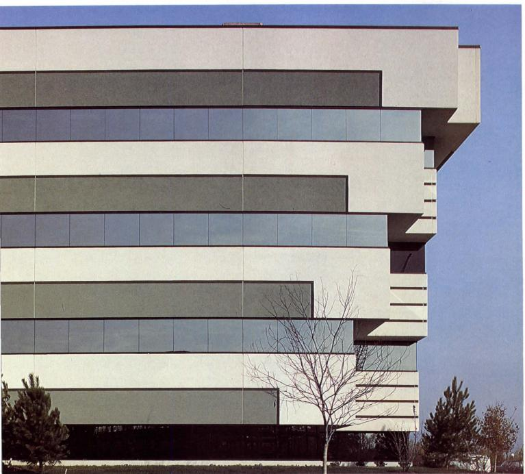
Belle Mead Building Architect: Henry Iggena STO INDUSTRIES, INC. Quality Lane, Box 219 Rutland, Vermont 05701 Toll Free: (800) 851-5533 Prefabricated Exterior Insulation Panel Systems
