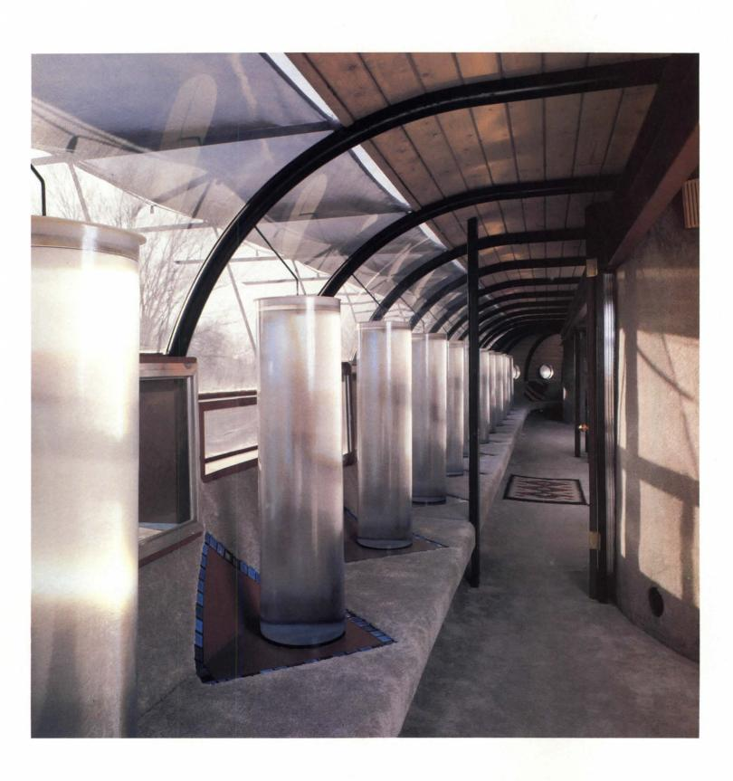
Structural steel I-beams support third-level bedroom quarters (below), which are clad in tongue-and-groove decking over custom-bent, three-inch-diameter metal ribs. By covering all walls and floors in monochromatic gray carpeting, Prince created a serene contrast to the more aggressive exterior—an effect that is heightened by light filtering through the translucent acrylic panels of a semicircular
