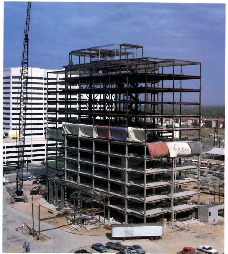
Vulcraft deliveries eliminated "lay down space" worries
