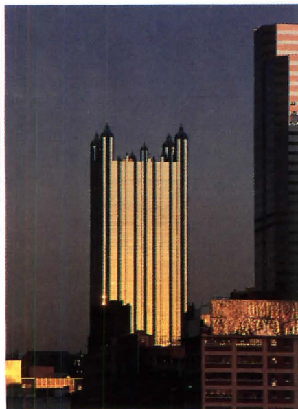
Like other reflective glass curtain-wall buildings, PPG Place visually responds to the varying ambient light of dawn, dusk, night, and full sun. Unlike other glass towers, PPG's "pleats" significantly extend its vocabulary of surface effects. At times, the Tower's monolithic form on the urban skyline is turned into a bundle of delicate, radiant shafts.
