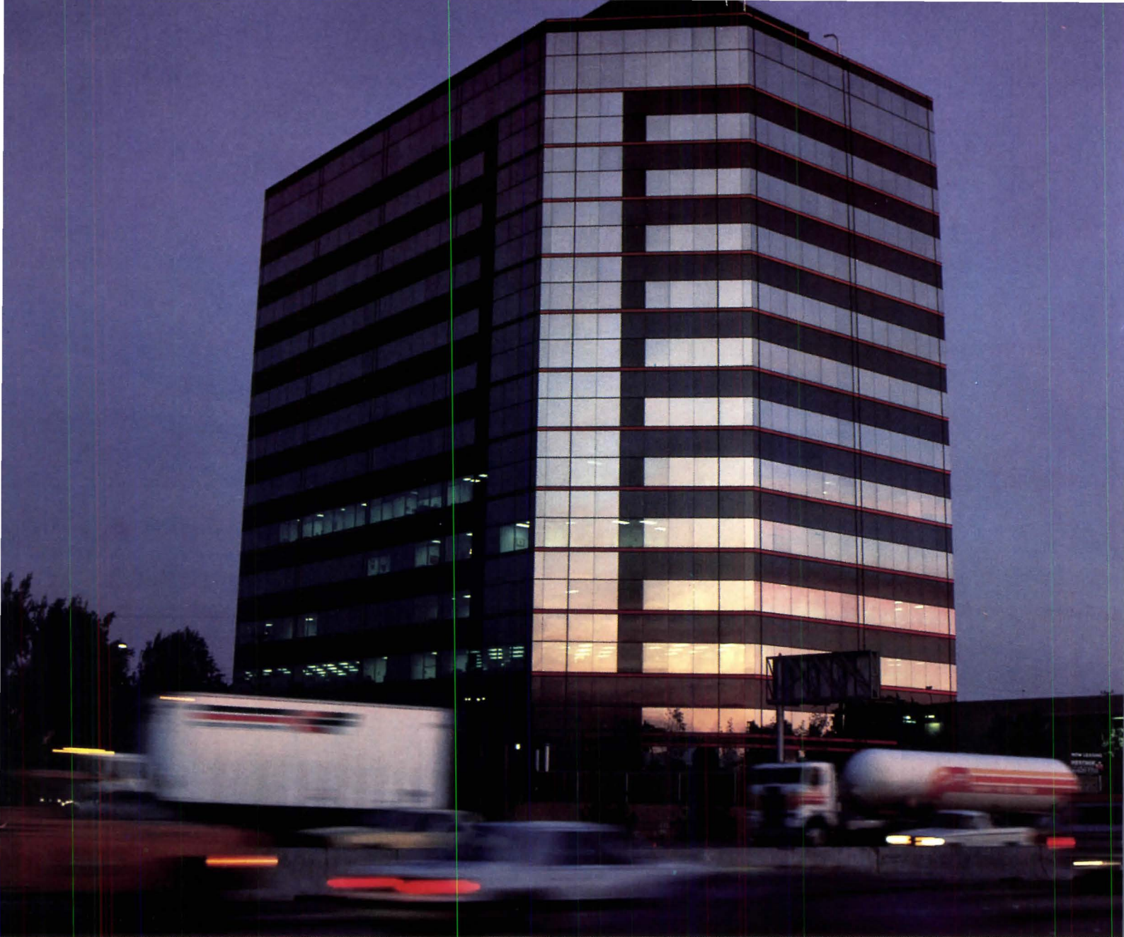
The Pepperdine University Plaza building was designed by Landau Partnership and is managed by Murdock Development Company.
