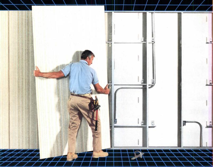
CB-350 is the most versatile, demountable gypsum partition system on the market today. The non-progressive GB-350 system provides immediate accessibility on either side of the wall at any individual panel location. The open stud design permits easy routing of utilities horizontally as well as vertically. Since wall panels are easily removed and replaced, you achieve maximum reusability for greater cost savings.
