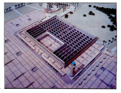
As the plan below indicates, the mosque is surrounded on three sides by an immense podium which is also the roof of a vast parking garage. Worshippers reach the podium by various flights of stairs from the parking and roadway level. VR&SB have placed the dome over the sahn (courtyard) rather than more traditionally above the mihrab (niche indicating direction of prayer toward Mecca). Thereby,
