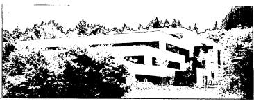
The three stories of Data I/O's manufacturing and office building step back in deference to the sloping site. On the side of the building, the main entry is at the lovest level (opposite and at top), from which stairs and planting rise to another entry at the middle floor. The 97,500-square-foot building cost \$44 per square foot.
