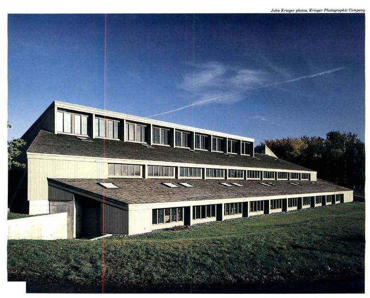
The tiered roofs of this DNA factory in Massachusetts attest the company's rapid growth. Phase I, 10,600 square feet completed in September 1979, included the clerestory and the middle floor shown above, and Phase II, 12,510 square feet completed in November 1982, included the lower extension and an angled wing at the southeast. A lounge at the end of the wing (opposite at top)
