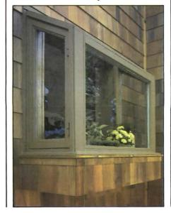
of fine-grained Ponderosa pine. This wood was chosen for its excellent insulating properties and the way it accepts a stainand-varnish, or paint, finish.
