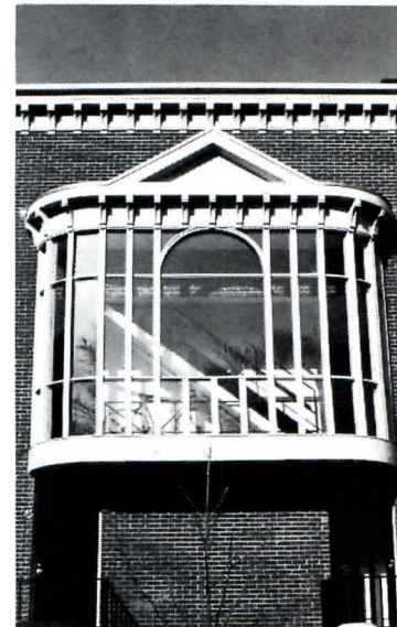
Wood oriel and fiberglass cornice, Georgetown University, Washington, D. C.
