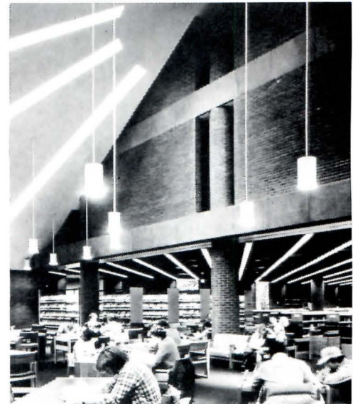
Return air plenum in reading room, Library and Learning Center, Gettysburg College, Pennsylvania
