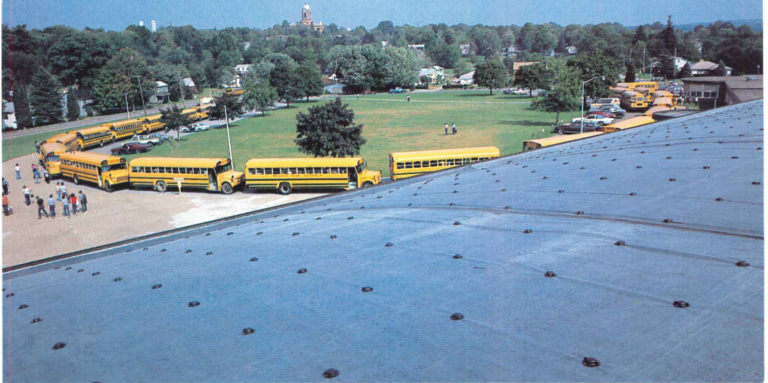
The Mercer Area High School, Mercer, PA Roofing Contractor: J.A. Burns & Sons, Mercer, PA
