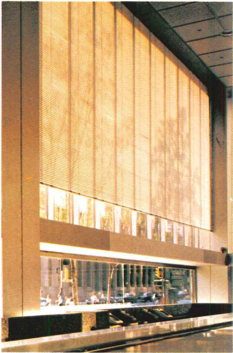
The Commerce Court in Toronto is comfortably lit with one of the world's largest banks of blinds, made by Hunter Douglas. They're electrically operated.
