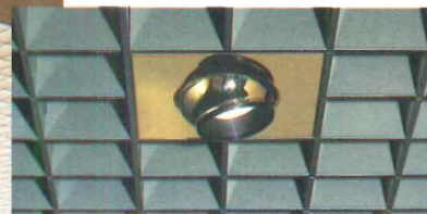
Reflector down lights – polished reflector, mounted for wall washing and overall illumination.
