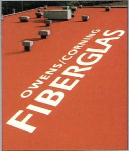
Perma Ply No. 28 base sheet. 2 plies Perma Ply No. 11. Perma Cap surface over wooden deck.
