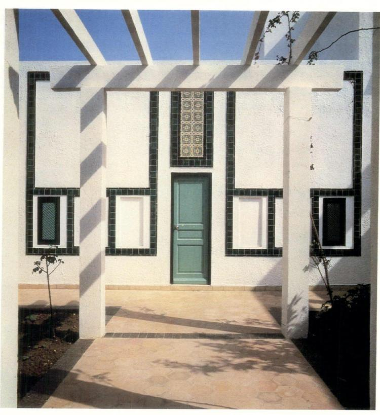
Bands of traditional tiles surround windows and form simple geometric patterns, not unlike those to be found on courtyard walls in traditional Arab houses. The windows are small and protected by wooden screens that filter the light. Doors are all of wood painted light green with dark-green frames. All joinery has been done by traditional methods.
