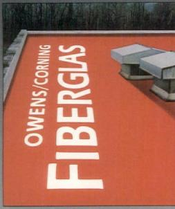
Double-layer Fiberglas insulation over FURI. 3 plies Perma Ply-R. Gravel surface.
