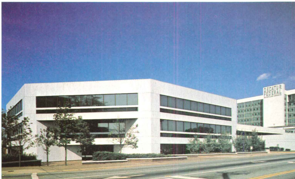
Decatur Federal Savings & Loan Assn. Building, Atlanta, Ga. Architect: Thompson, Hancock & Witt Associates, Atlanta, Ga. Stone Setter: Williams Tile & Terrazzo Co., Smyrna, Ga.
