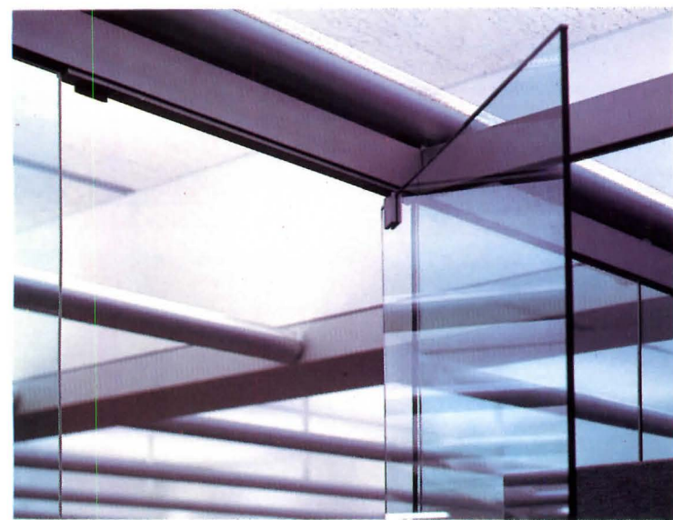
A view of one bay of the mock-up (above) shows the relationship of the transparent perimeter private offices to the interior work stations. The uplight reflected from the concealed-spline acoustic-tile ceiling has a pleasant, slightly-perceptible modulation which, with the transparent partitions, helps create the open feeling desired by the company. The 22-ft-long light tubes have one hanger in the center to control deflection. The indirect light from the tubes, fitted with cool-color, high-color-rendering lamps, complements the daylight from the windows. Evenness of the lighting has functional as well as esthetic attributes since it offers glare-free illumination for use of the CRTs. The system meets the Connecticut energy-code requirement of 1.6 watts per square foot. The outer three fixtures can be switched by a programmed light-control system.
