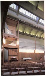
The congregation may face either north (directly above) or east (opposite); religious furniture and the cross are transposed to the appropriate wall as orientation demands. Shaped laminated wood arches support the vaults, which arches support the values, which are planked with pale stained yellow pine. Concrete struts, which transfer load from the top vault across the clerestories to the side walls, were known by the construction crew as angel wings.
