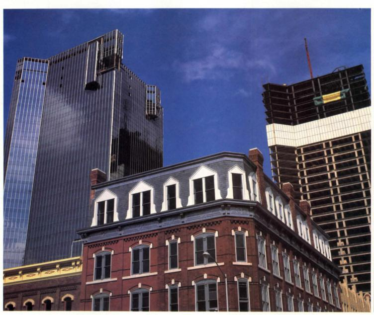
Exposed tripod and clustered-pair columns are scale-relating elements for Tower 1 (left) and Tower 2 (right) in City Center, which also embraces two blocks of historic building renovation (foreground) by the same developer. Rudolph expressed the plasticity of the curtain wall with turrets at top and bottom and wings at corners, and he notched Tower 1 to admit daylight to a skylight.
