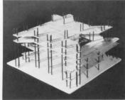
Rudolph built structural models for the owner and the engineer to clarify column relationships. The architects, engineers, and contractor, in fact, used the models to garee upon column positions for locating foundations.
