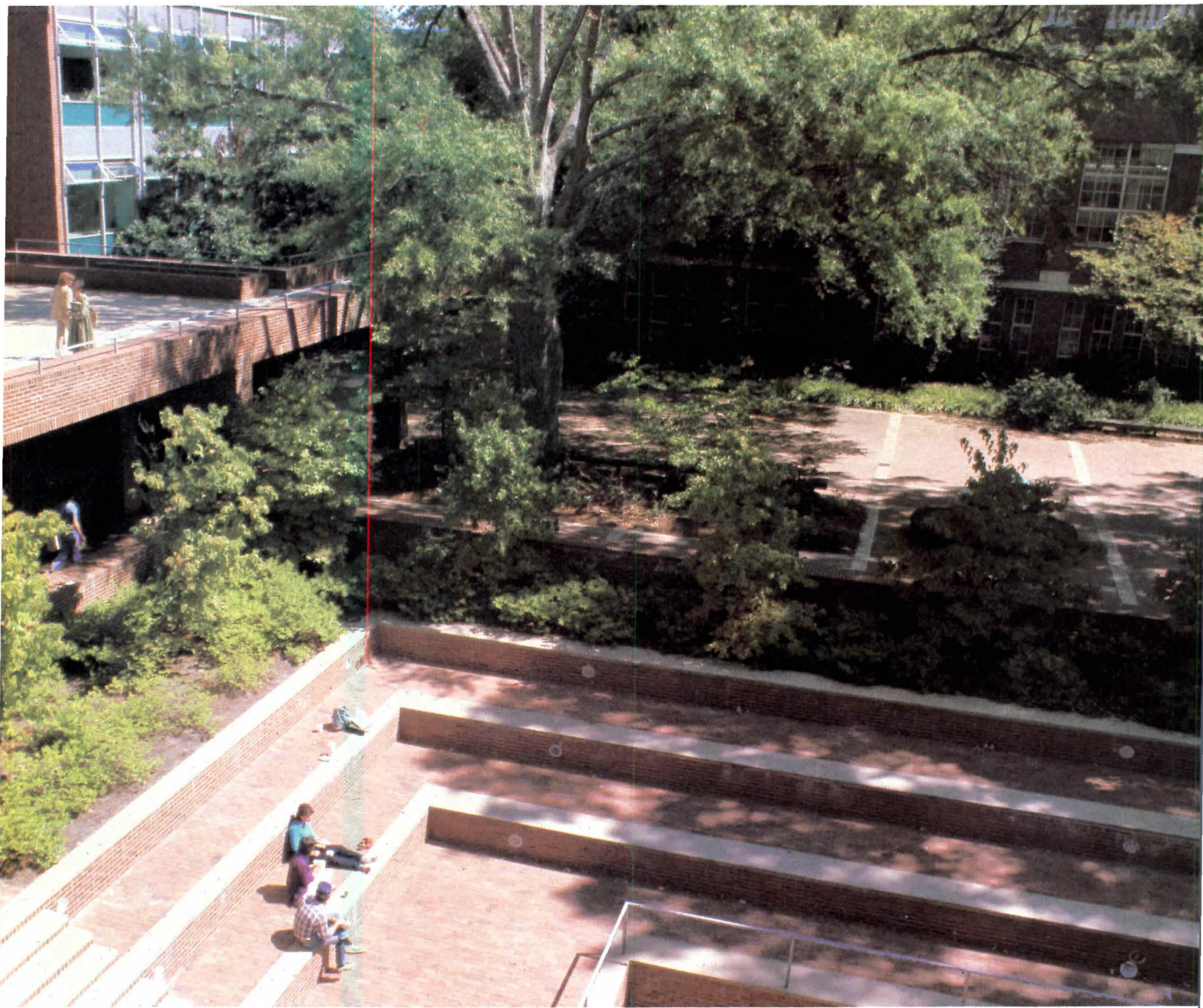
NORTH CAROLINA STATE UNIVERSITY SCHOOL OF DESIGN ADDITION
