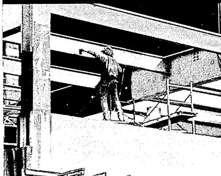
Penthouse Casino, Atlantic City, N.J. Consulting Engineer, DeSimone & Chaplin Assoc.
