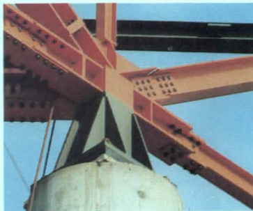
Steel box sections embedded in 5-ft-high column caps are bolted to the space truss with 3-in.-diam anchor bolts. Four-foot-square elastomeric pads accommodate rotation at each connection.
