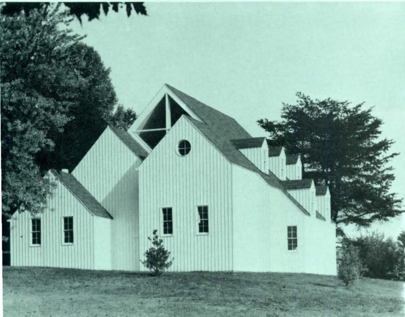
3 Hartman-Cox Architects photo
