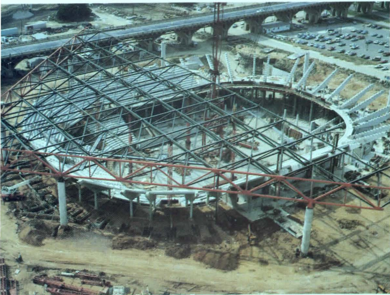
The Arena's 176,400-sq-ft space truss is supported on eight 6-ft-diam columns. The roof has a 412-ft clear span and overhangs the substructure by 4 ft on each side. The frame's corners cantilever 70 ft from the column line.
