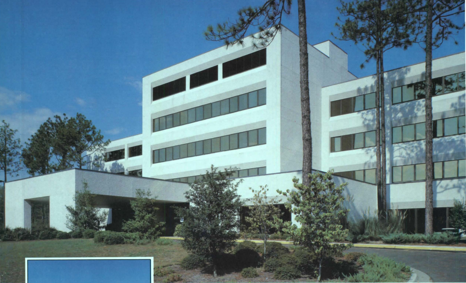
Aiken Community Hospital Aiken, SC - Architect — Gresbam & Smith
