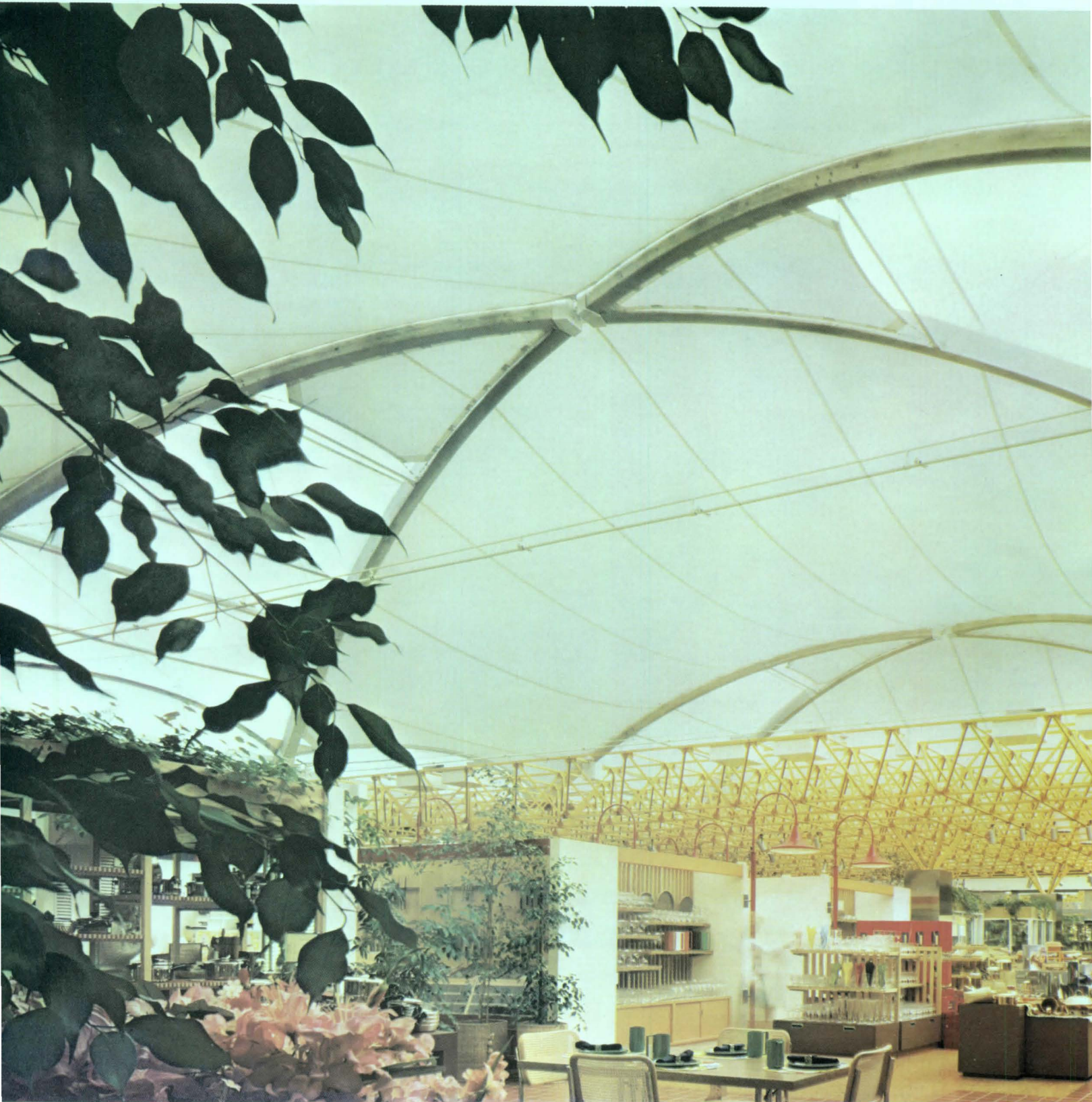
Bullock's, San Jose, California—the world's first department store under a permanent Owens-Corning Fiberglas fabric structure. Environmental Planning and Research, Inc., architects and planners. Geiger-Berger Associates, structural engineers.
