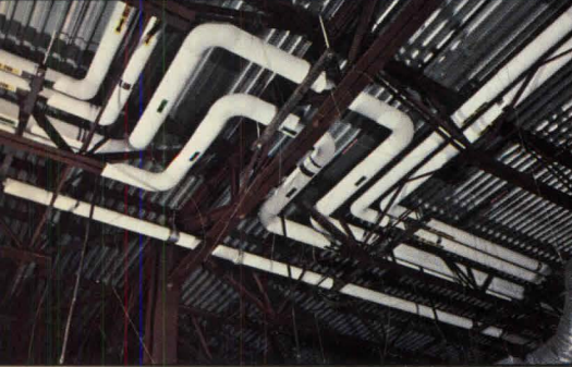
Because electrical and mechanical systems can pass through the open web of the joists and joist girders, installation goes quicker. And changes can be made more easily when needed.
