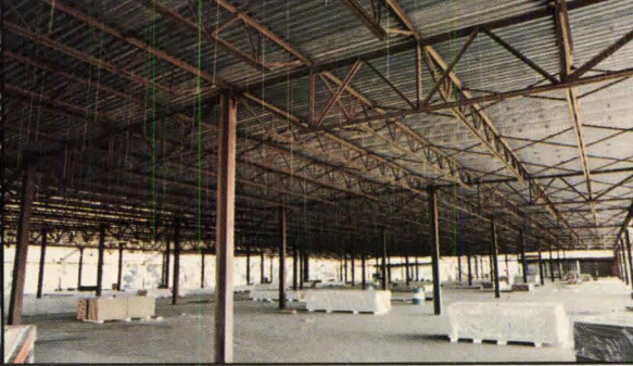
The high strength to weight of steel joists and joist girders can provide increased clear span areas, because supporting columns can be spaced further apart.
