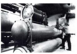
**INDUSTRIAL HEAT PUMP** / A nonreversible heat pump/water heater capable of recovering industrial or hvac waste heat in commercial and industrial buildings and amplifying it to temperatures up to 220 deg. F, the *Templifier* water-to-water pump can provide economical heat for process fluids, make up water, and hot service water in offices and institutions. • Westinghouse Electric Corp., Staunton, Va.
