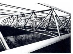
LUMINUM TANK COVERS / Pre-engineered aluninum roofing systems are specifically designed to over large tanks where long spans are necessary. ow-profile design, with or without headroom, ncorporates access hatches or walkways. Tank overs are bolted together on-site from lightveight, corrosion-resistant components; roof cladling may be enameled or stucco embossed aluminum sheet, or fiberglass or acrylic panels where ght transmission is required. • AEF Aluminum tructures Ltd., Scarborough, Ont.
