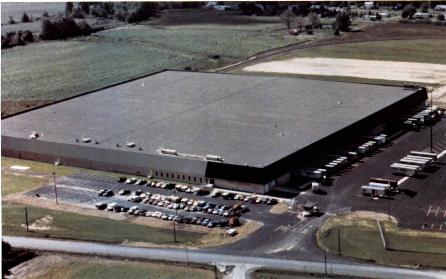
Aerial view of the Carlisle roof on the new Milton, Pennsylvania Distribution Center built by Weis Markets, Inc.
