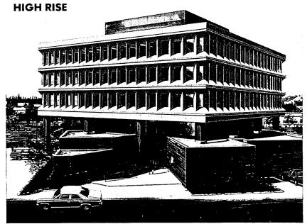
The permanence and appearance of pre-cast concrete at oneeighth the weight. Window wall unit was glazed and insulated in the factory offering substantial cost savings at the job site. Insulation was installed within the panel without any loss of floor space. Architect: Simpson, Usher, Jones, Inc., Anchorage, Alaska. Manufacturer: Olympian Stone, Redmond, Washington.
