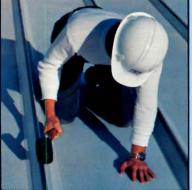
Panel seams are locked into position by striking along the seam length with a rubber mallet (no crimping devices or sealing machines). Clips hold panels to purlins.
