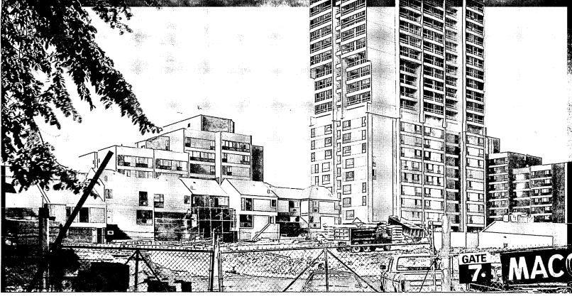
The townhouses are woodframe construction with brick and wood shingles as the exterior material. They are being constructed over a 1,274-car underground garage of precast concrete. Available to all the residents in the high-rise, midrise and townhouses are dishwashers, disposals, a swimming pool, tennis and basketball courts, six play areas for small children, a formal plaza with a fountain and extensive landscaping.
