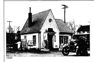
(21) The malleability of the vernacular building shell is illustrated by this almost unbelievable example of the expansion and transformation of a small traditional gas station into a modern one, complete with corporate logos and standardized details. The remodelling of this Mobil station occurred in the early 1930s, and a drawing showing the "before" and "after" conditions is shown below.
