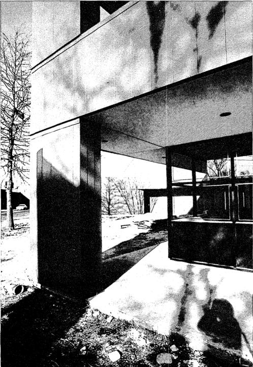
These details show that "industrial" materials often used badly can take on real distinction with careful attention to the real capabilities of the materials. This garage building-sheathed in a stock curtain wall-has the character of a sculptural construction. The translucent fiberglass panels and steel wall panels are mounted in aluminum frames and are factory finished on both the outside and inside.
