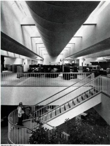
Light level on the upper floor reaches 200 fc of glareless illumination on a clear day, without assistance from fluorescent lamps installed below skylight for use on gray days. Double glazing is reflective outside, unpolished glass inside. Daylight is reflected off gypsumboard facing on girders and off the deep catenary curves of the "socks." Library (lower left) is one of the building's few partitioned-off spaces.
