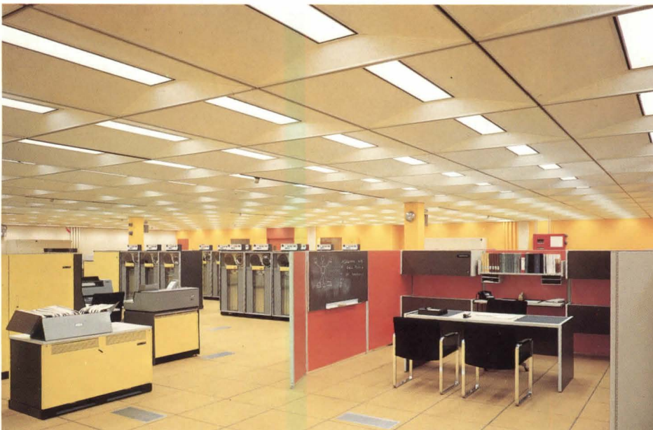
Datacenter/The Equitable Life Assurance Society of the United States, Easton, Pennsylvania, Architects: Kahn and Jacobs, New York City, Ceiling System: Armstrong C-60/60 Luminaire
