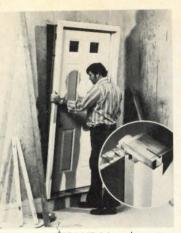
TEEL DOOR<sup>†</sup>FRAME / A prehung resdential exterior steel frame, *Perma-Trame* installations need no brick nold finishing. When combined with a steel *Perma-Door*, the entry is said to offer excellent home security. The allteel assemblies have synthetic rubber weatherstripping; the door botom/threshold seal passes the ASTM water and air infiltration test. • Steelcraft Mfg. Co., Cincinnati, Ohio.
