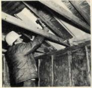
**ROOF VENT** / Designed to provide necessary air ventilation from soffit to attic, 48-in.-long *Proper Vents* are stapled to the underside of roof sheathing at the cornice and plate line. Each vent provides a 16-sq-in. air space to control attic moisture and prevent ice buildup and damming on the roof. • WaynRoy, Inc., Minneapolis, Minn.
