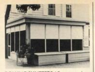
ROLLING SHUTTERS / Energy savings and increased residential security are claimed for these vertical rolling shutters, installed on windows, doors, screened porches, etc. Each PVC plastic slat is an extruded double wall with a dead-air space, said to act efficiently as a sound and thermal barrier. Once lowered, the shutters can be locked from the inside; the slats can be adjusted for any degree of light control. • Ever-Strait Door Systems, Fairfield, Ohio.
