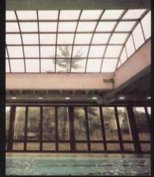
This skylight is representative of the type of skylights now being fabricated with "Lucite" cast acrylic sheet.
