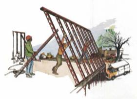
Structural components included in Inryco/Milcor steel framing systems can support the entire weight of buildings up to five stories high. Components are frequently pre-assembled for installation in large sections to save construction time.
