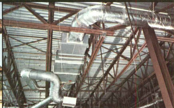
Vulcraft joists and joist girders can be designed to easily accommodate all lighting, heating, air conditioning, wiring, duct and pipe requirements.
