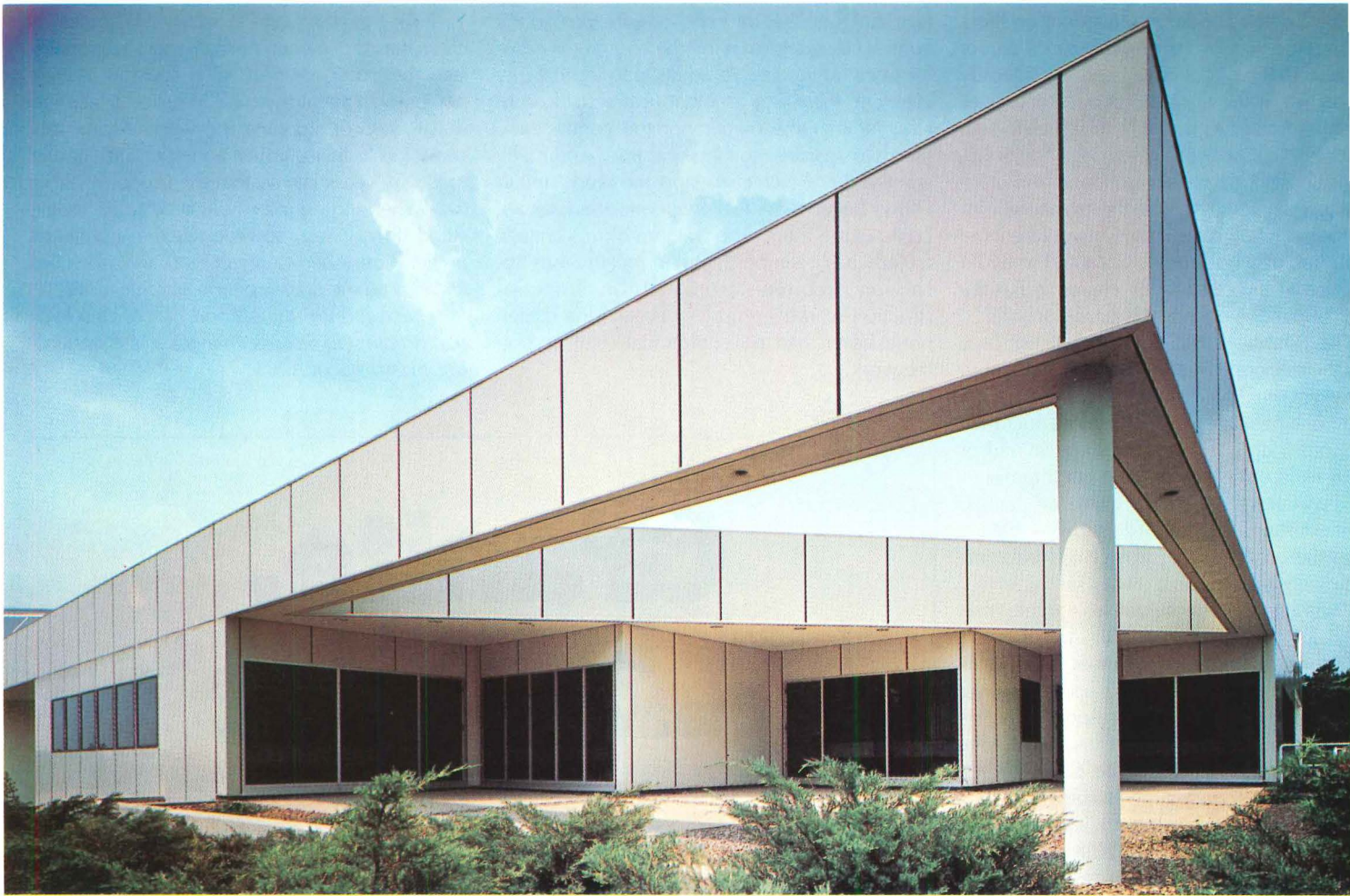
Project: Coastal Industries Office Building, Bath, Ohio Architect: Perkins & Will, Washington, D.C. Curtain Wall Erector: Handcraft Metals Corp., Cleveland, Ohio
