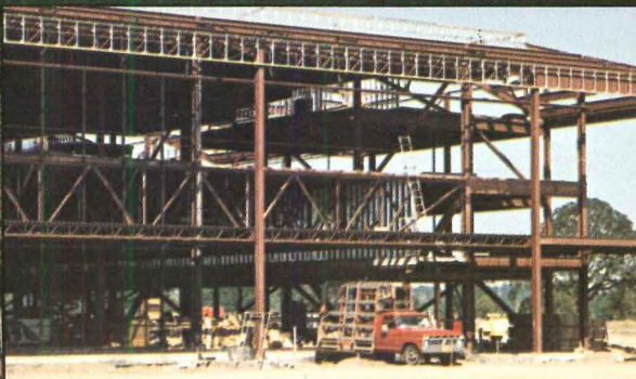
The versatility of designing with Vulcraft steel joists and joist girders helps meet complex design requirements like this unusual eight foot interstitial floor space.
