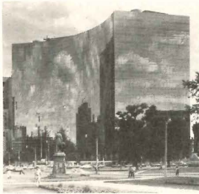
Aerofin Types C, CB/R, RC Cooling Coils were used in HYDRO PLACE, new Toronto headquarters of Ontario Hydro.
