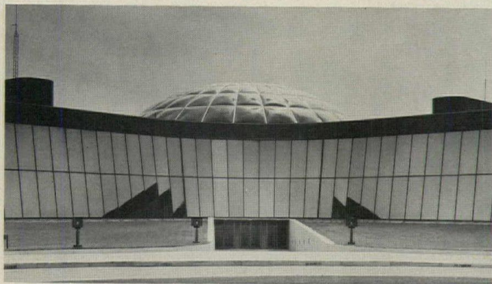
BRYANT COLLEGE Smithfield, Rhode Island (Exterior)
