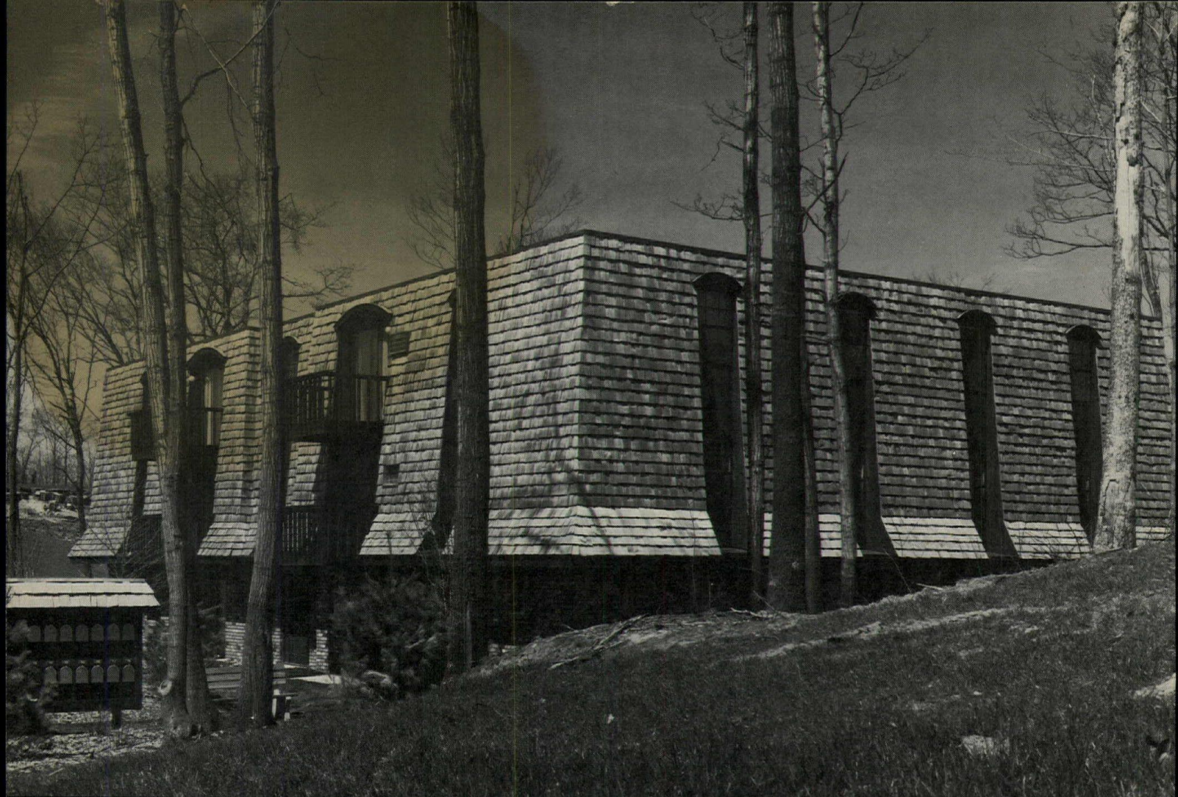
Glenbrooke at Century Hills Apartments, Rock Hill, Connecticut. Frazier & Vigneau, Architects.
