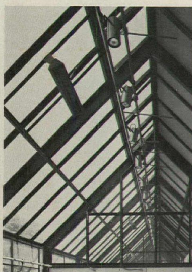
SUFFOLK COUNTY COMMUNITY COLLEGE Fine Arts and Classroom Building, Selden, New York
