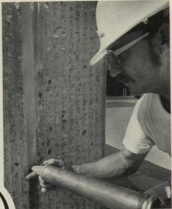
Applying an LP® polysulfide-base sealant.
