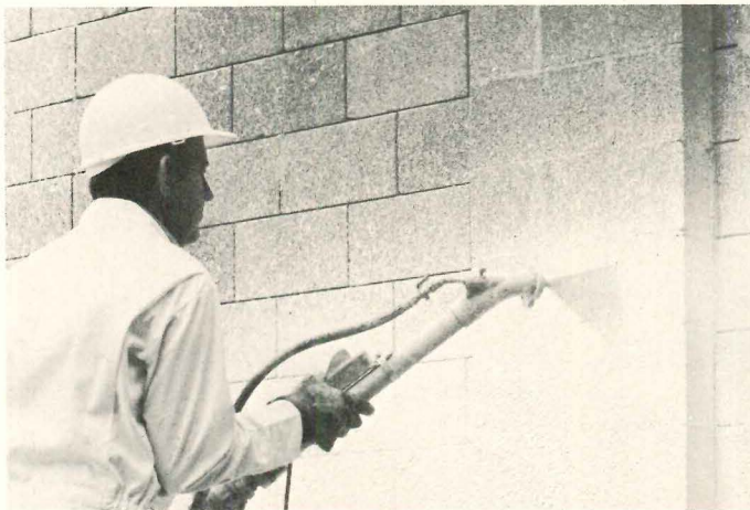
Spraying is the fastest way to apply BlocBond. Three men can cover about 1200 sq. ft. an hour.
