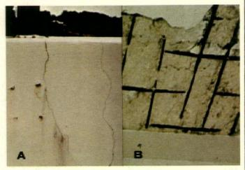
The rusting of ungalvanized reinforcing bar creates a pressure which can crack and spall concrete. Photo A shows a portion of the facade of the Charleston, S.C. Post Office which has been cracked and stained by subsurface rust expanding and "bleeding" through. Photo B shows the underside of a veranda roof in Bermuda where rebar corrosion caused a large section of concrete to fall off.
