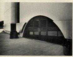
Because all levels that open to the atrium can be exposed to a single fire emergency, the evacuation plan was based on simultaneous exiting of all occupants. Doors at the bottom of the enclosed stairways open directly to grade. Stairways are pressurized by fans in the event of fire. All office areas are fully sprinklered, and a gravity venting system was designed to draw smoke from the atrium and also from the area involved if a fire occurs.
