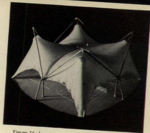
Figure 16: four-tent configuration for tennis courts
