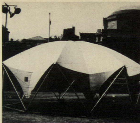
Figure 5: a frame-supported tent experiment
