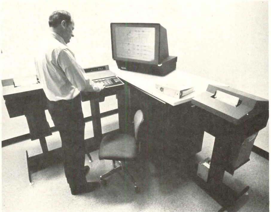
Automation control center in the Health Sciences building now handles a 10-building complex.
