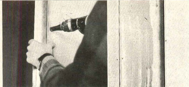
3. Attaching core to T-spline.
