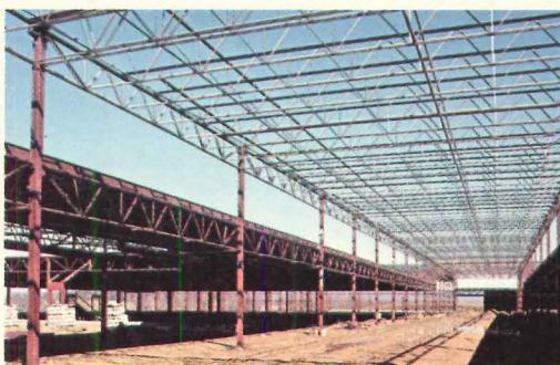
The high strength of steel joists and joist girders provides increased clear span area, allowing larger bays.
