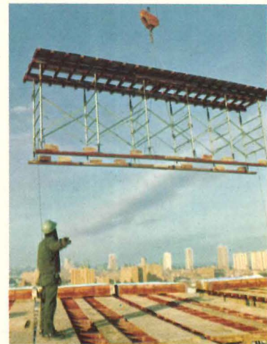
Montgomery Ward Corporate Offices, Chicago Architect: Minoru Yamasaki & Associates Structural Engineers: Skilling, Helle, Christiansen & Robertson General Contractor: Turner Construction Company Concrete Contractor: S. N. Nielsen Company
