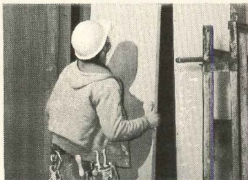
2. Installing core panel.
