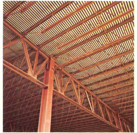
Joist girders have top chord panel points that show joist location. Which makes a lot of measuring unnecessary.
