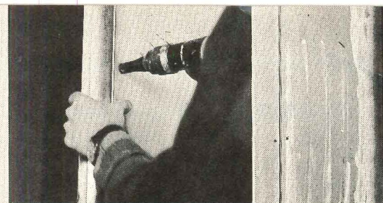
3. Attaching core to T-spline.
