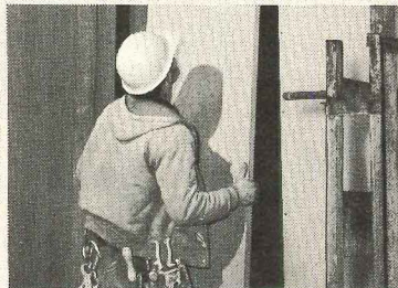
2. Installing core panel.
