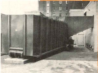
Through-the-wall loading into a Dempster Packer provides a convenient, all-weather refuse disposal system.
