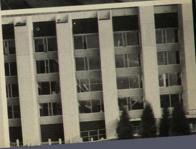
All services to the laboratory benches (left) are delivered from exposed piping in the ceiling which passes through perforations in the precast structural girders. The exhaust ducts at the rear of the laboratory wing (right) are five-stories high. At this point in-line fans expel the fumes. Ten of the 15 shafts are heavily used and five lightly.
