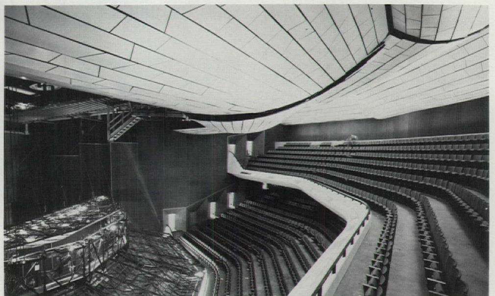
Figure 18 Over-all view of the auditorium with all house lights on, showing the movable ceiling from the rear in the intimate drama theater configuration. Cut-off of the remaining volume of the auditorium demonstrates conclusively how the continental seating system of side aisle access only (with all houselights behind lowered portions of the ceiling turned off) allows the auditorium to be reduced in size without the audience being aware either during ingress, egress, or when seated in the auditorium or moving about in the lobbies that the reduction in size is at all a makeshift architectural arrangement.
