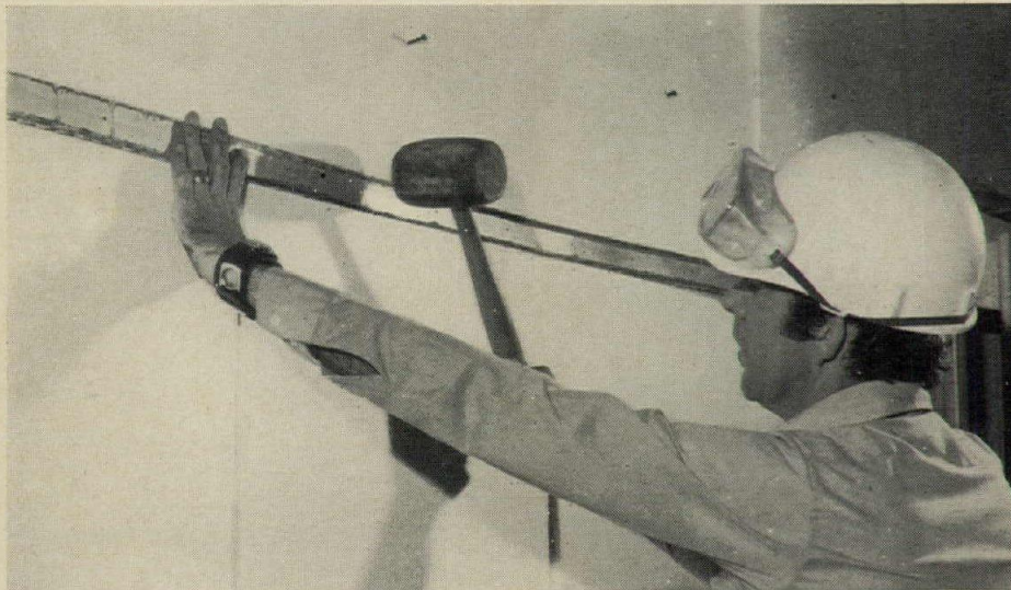
Imbed THERMO-STUD channel in Foam.
