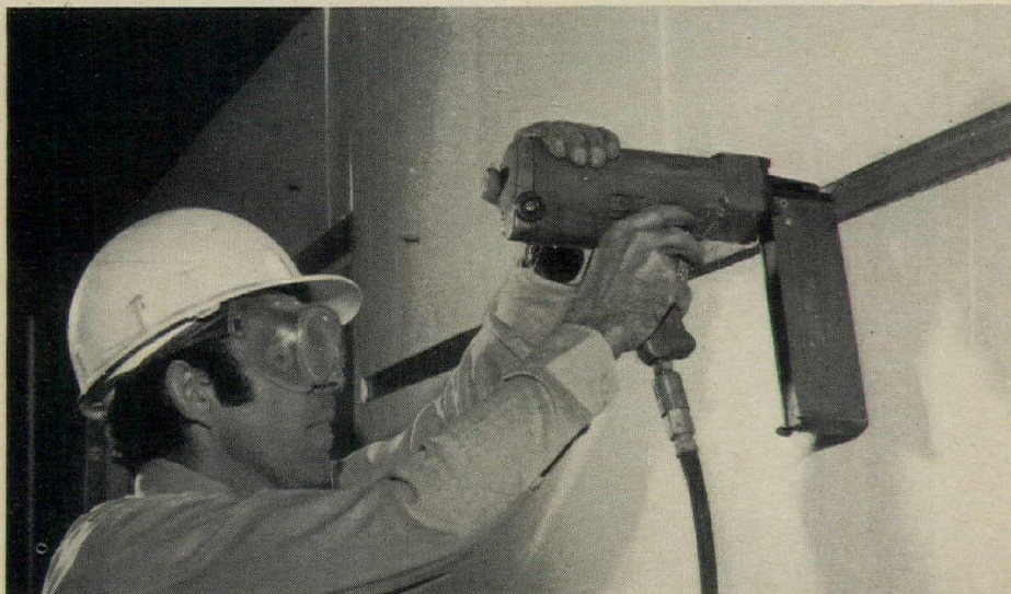
Nail through Foam to masonry.
