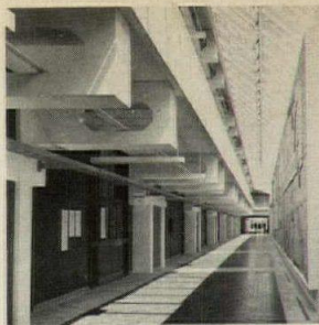
Cover: Undergraduate Science Center Harvard University, Cambridge, Massachusetts Architects: Sert, Jackson and Associates, Inc. Photographer: Steve Rosenthal
