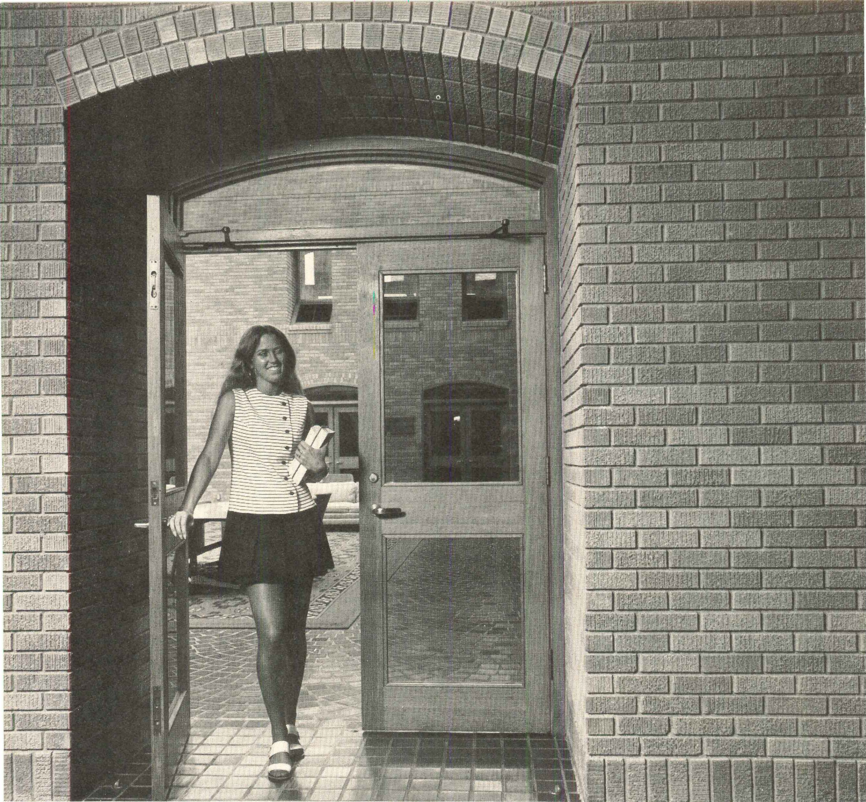
Texas Tech Law Building, Lubbock, Texas. Omniplan Architects Harrell & Hamilton, Dallas.
