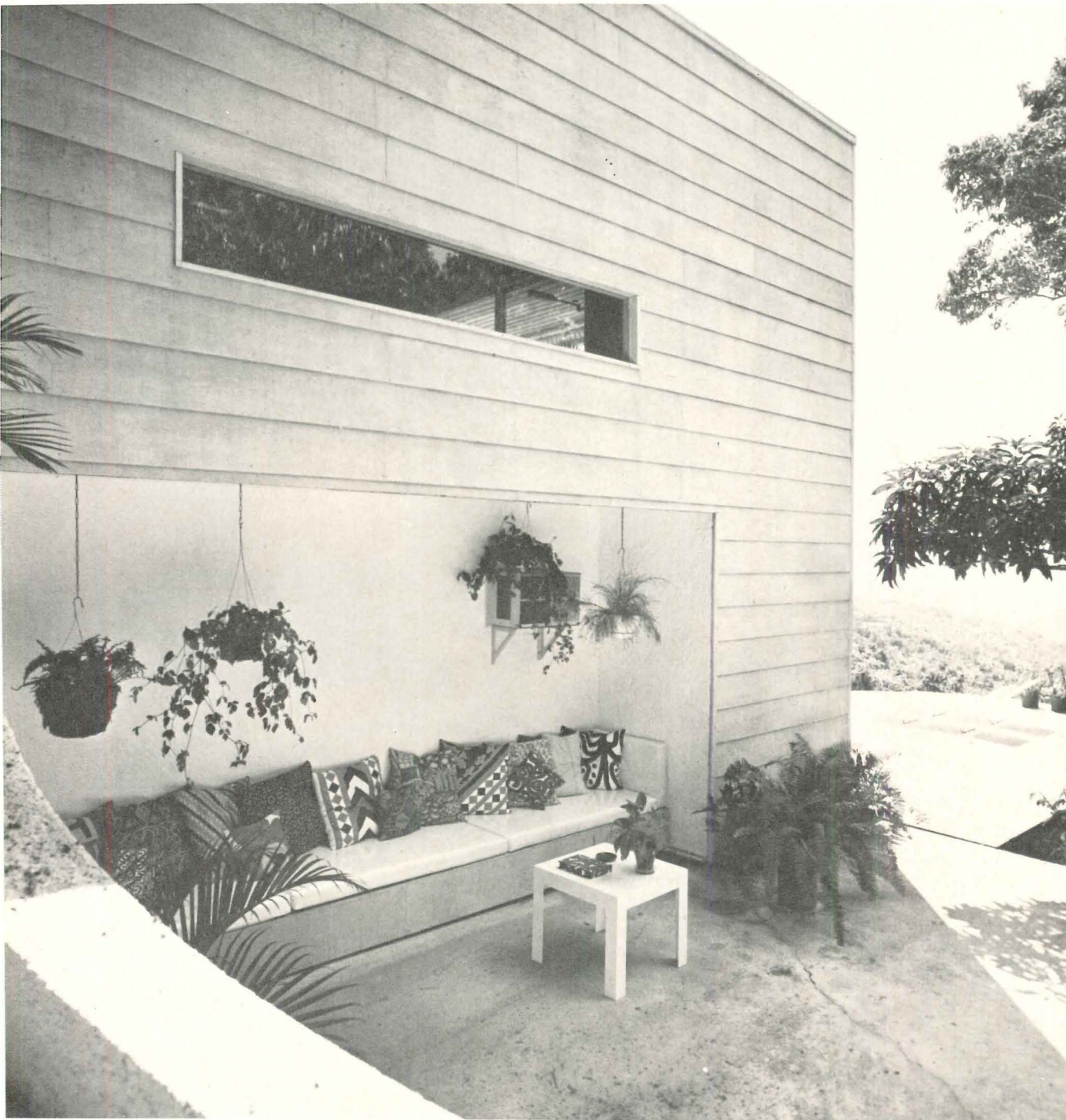
On the north side of the house, at right angles to the direction of the slope, Bates has developed a small terrace protected from the sun. The master bedroom (photo right) with a strip window over the headboard, overlooks the terrace and opens, at the side, into a covered gallery.
